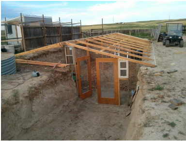
The outer dimensions are 24'x40' The rafters span 2' over the ground on all sides of the walipini.
