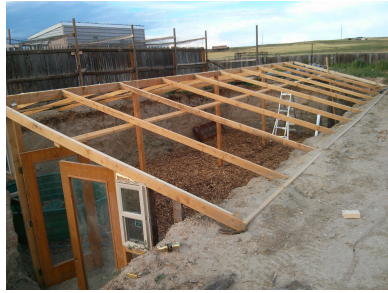
The outer dimensions are 24'x40' The rafters span 2' over the ground on all sides of the walipini.
