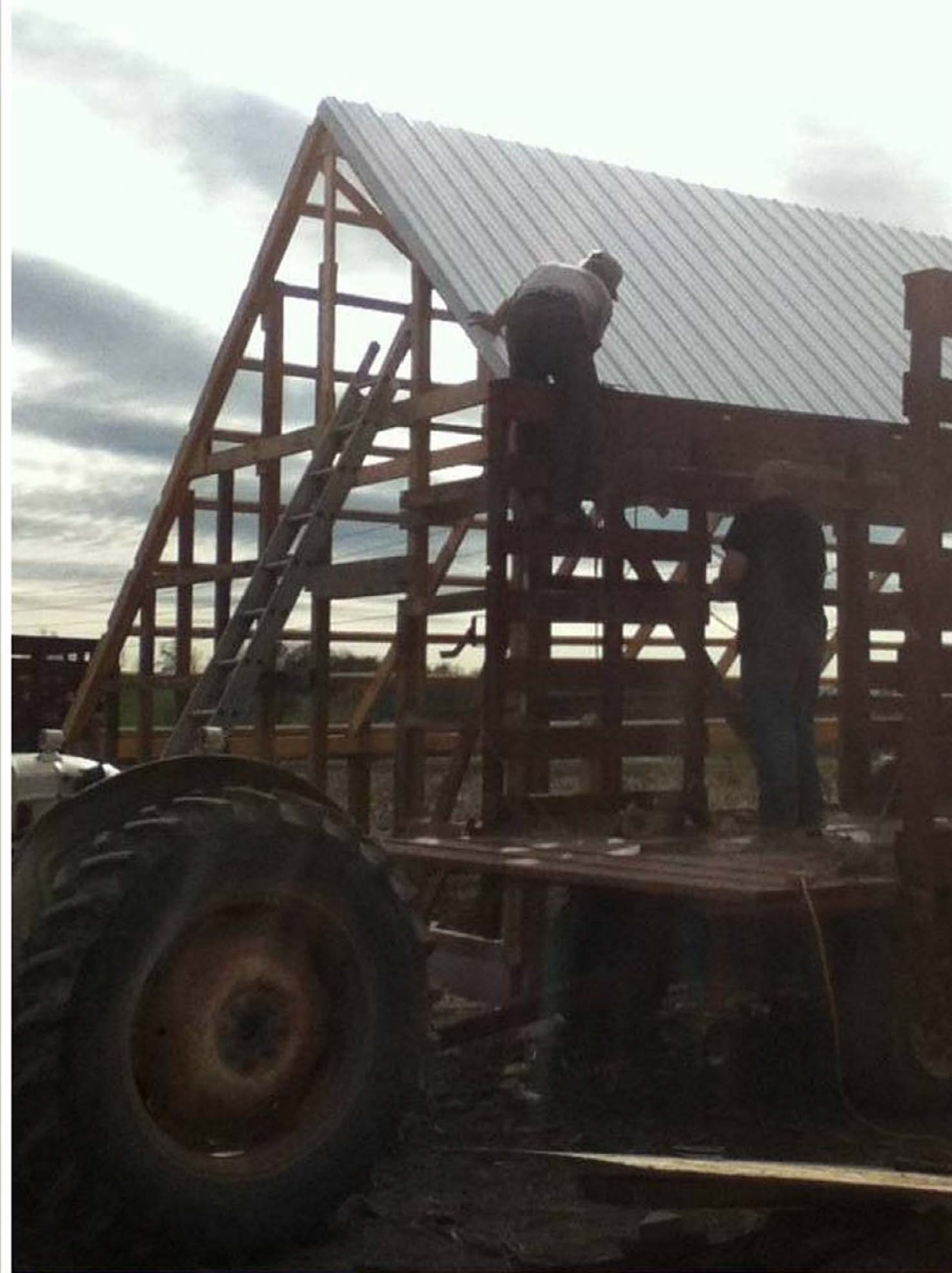
b finishing the roof
