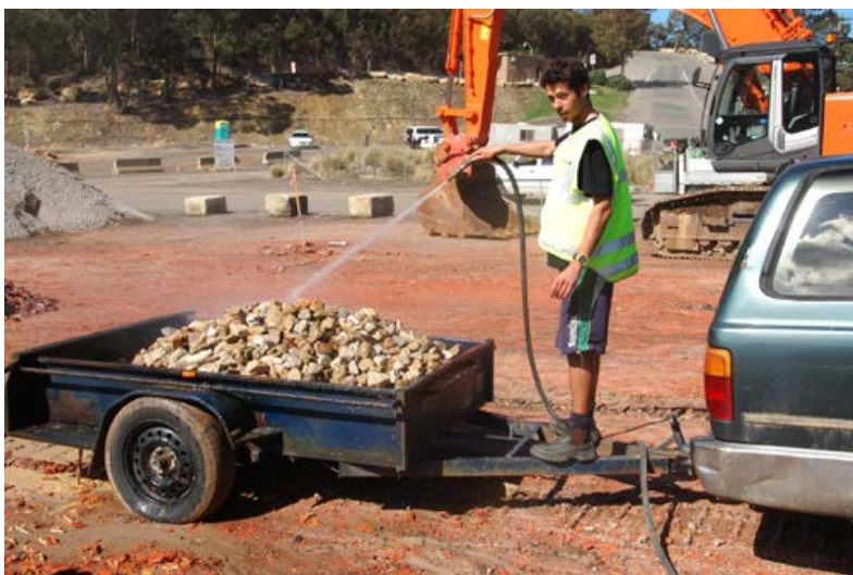
"how much weight did they say this trailer could take?" Jason "not sure, a trailer load? we will be driving very slowly" me (note: mud guards on trailer) Pre-rinsing gravel with onsite dam water. We eventually had to hand scrub every rock individually to remove the clay, close to a tonne.
