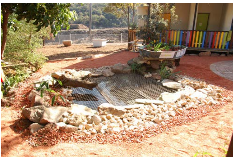
Pond the day after completion
